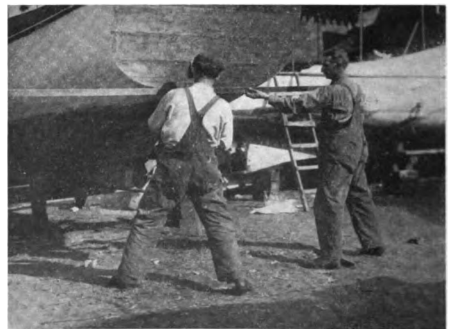
Raising the Water-Line
